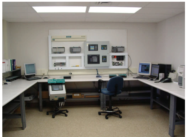
Figure 4. PLC Development Area
