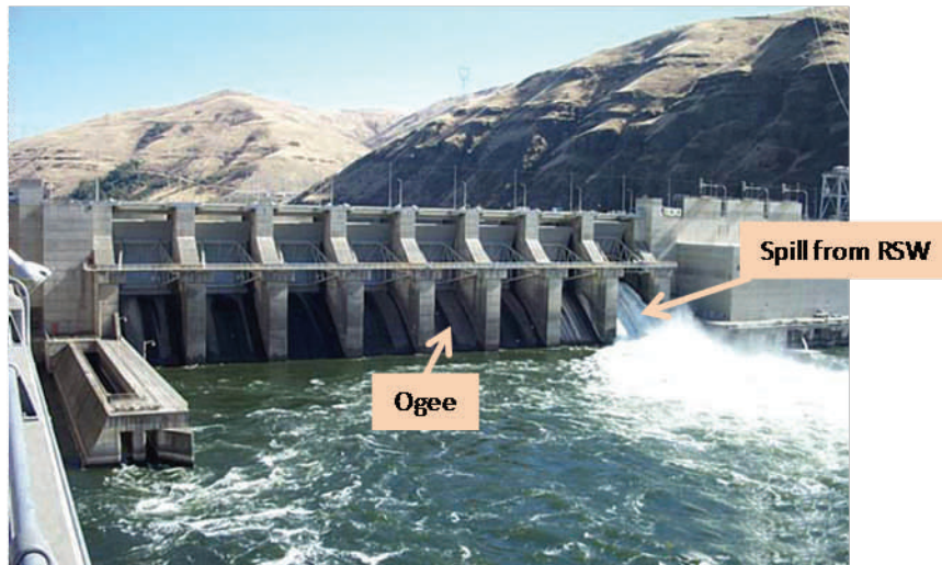
Figure 2. Photo of the spillway at Ice Harbor Dam with spill coming out of the RSW Spillbay and the ogee area marked for one of the spillbays.
